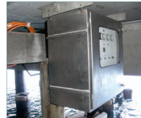
Typical CP Transformer Rectifier Unit
