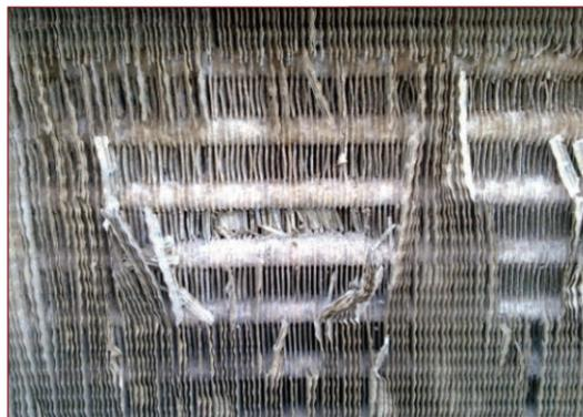
*Corroded coils due to salt and pollution.*
