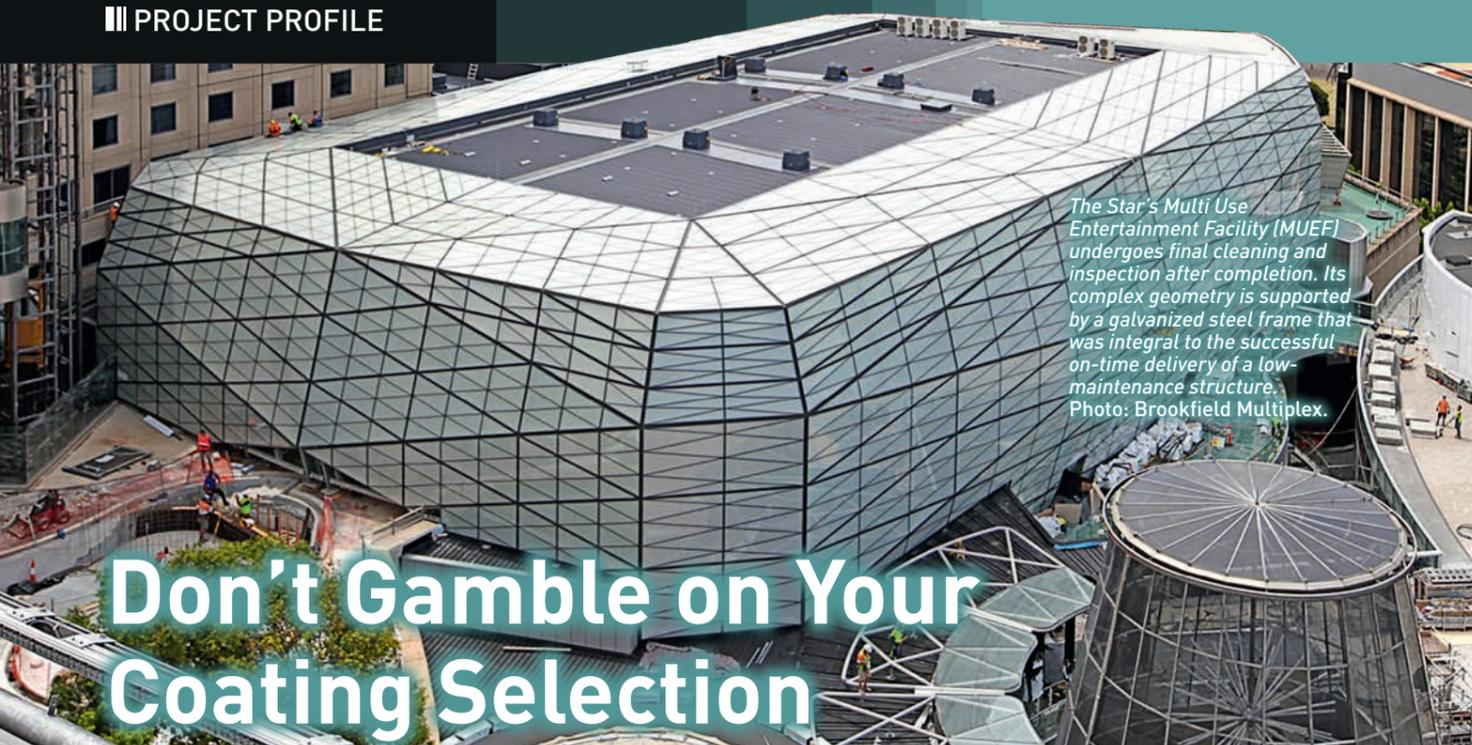
The Star's Multi Use Entertainment Facility (MUEF) undergoes final cleaning and inspection after completion. Its complex geometry is supported by a galvanized steel frame that was integral to the successful on-time delivery of a low-maintenance structure. Photo: Brookfield Multiplex.
