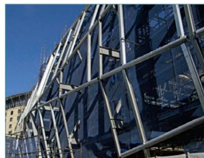
The MUEF during final construction phase; the internal sound-proof walls are in place, the stainless steel framework has been fixed to the HDG steel and the first glass panels have been installed. Photo: Industrial Galvanizers.
