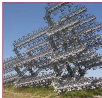
The Desiring Machine is a public artwork made entirely of galvanized steel. Weighing approximately 50 tonnes, the structure is 36 metres long, nine metres high and eight metres wide. The corrosion protection of galvanizing will ensure that it has a long lifespan with a minimum requirement for maintenance.
