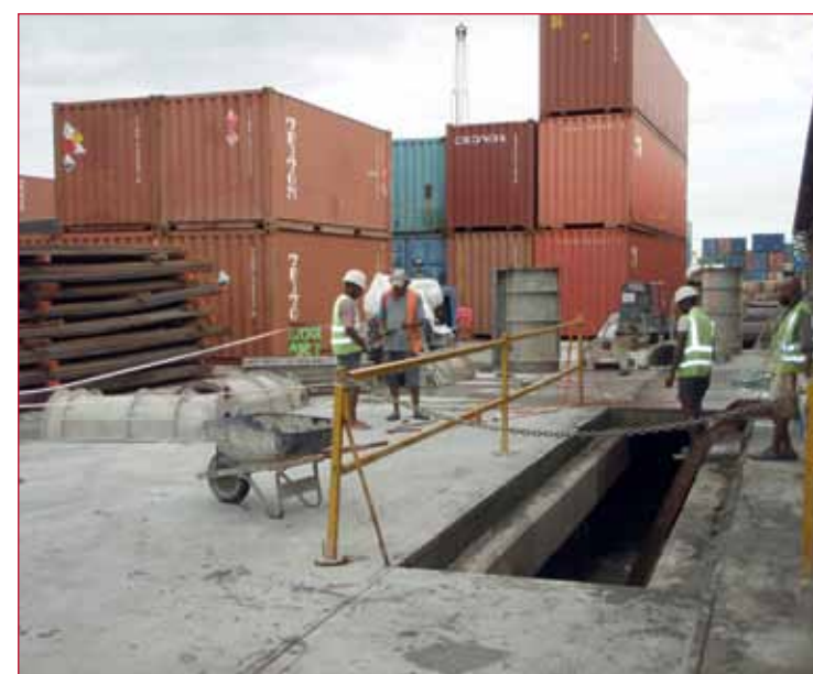
Access was required to the soffit of the wharf
