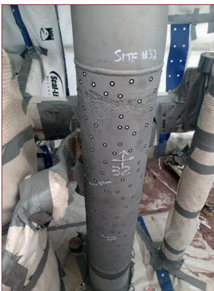
Figure 1. Cold shoe (pipe support) has been removed and the pipe has been cleaned and is ready for scanning.
