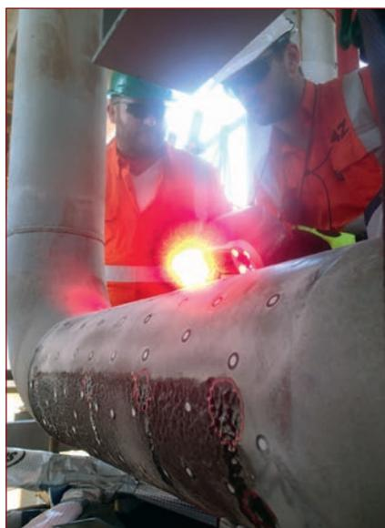
Figure 2. 3D data acquisition of the corroded area.
