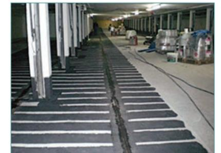
Figure 4 : Zebra conductive coating on a floor slab before application of high build cementitious overlay.
