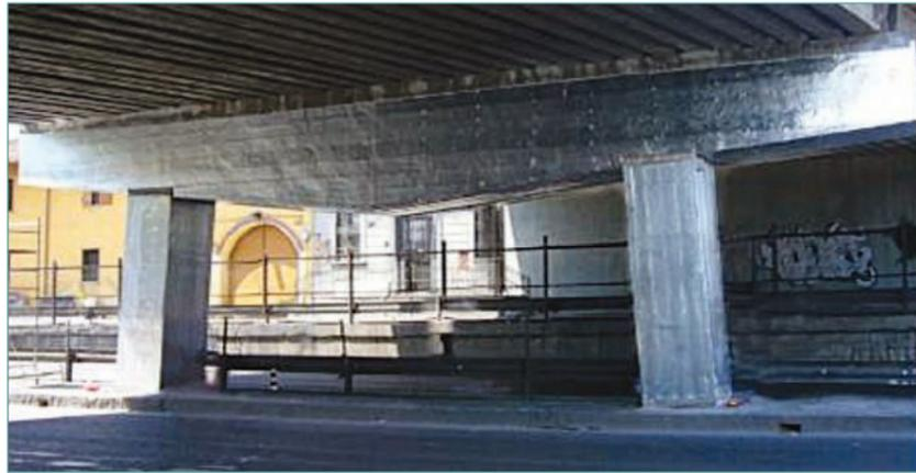
Figure 1 : Zinc Layer Anode applied to bridge beam and columns prior to application of top coats.
