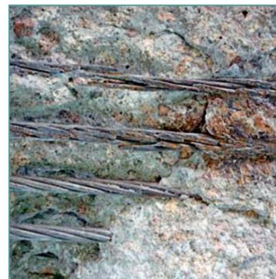
Figure 2. Typical chloride induced deterioration of the prestressed concrete beams.
