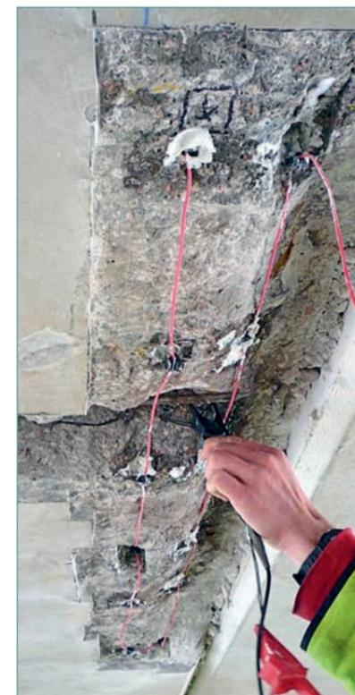
Figure 3. Typical hybrid anode installation on a prestressed concrete beam.
