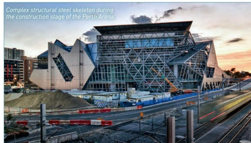
Complex structural steel skeleton during the construction stage of the Perth Arena.
