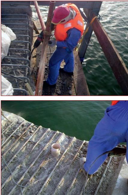
Figures 2 & 3: Impacting Method - Removal of deteriorated concrete by jack hammer.
