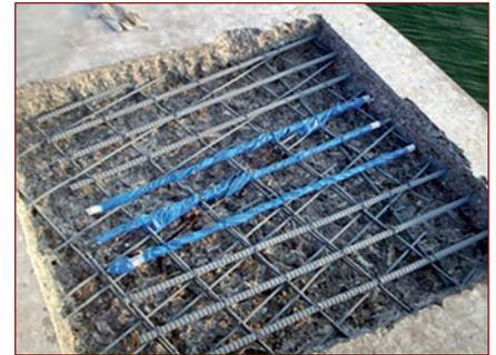
Figure 5: Steel cleaning and splicing by lapping after removal of concrete.
