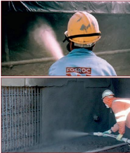
Figure 6: Sprayed repair mortar application .
