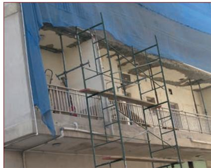
*Repair of balcony concrete corrosion and spalling due to multiple factors.*
