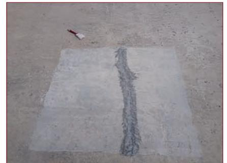
Surface grinding to open the face of the crack and sealing with epoxy resin.
