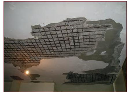
*Soffits severely corroded due to roof leakage into a residential building.*
