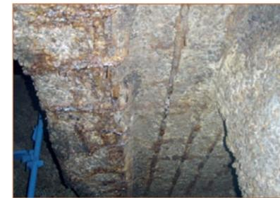
Photo 4 – View of the underside of a concrete platform within the drop structure prior to repair.
