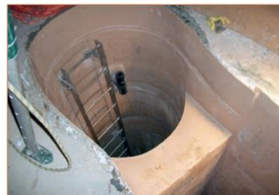
Photo 3 – Sewerage manhole after rehabilitation utilising mechanically anchored HDPE liner.
