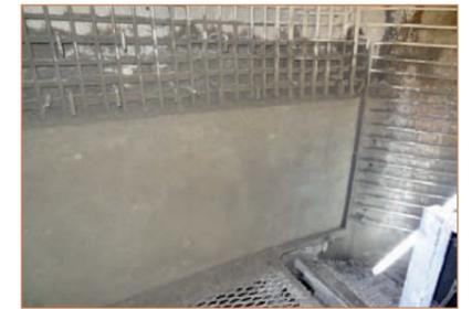
Photo 7 – View of wall within the drop structure being reinstated using a dry spray applied CAC.
