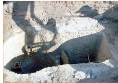
Photo 2 – Sewerage manhole following removal of the top slab and before rehabilitation.
