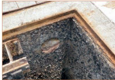
Photo 1 – Photograph of an un-protected concrete waste water structure showing initial signs of concrete degradation.
