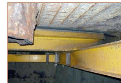
Photo 6 – View of the underside of a concrete platform within the drop structure prior to repair.
