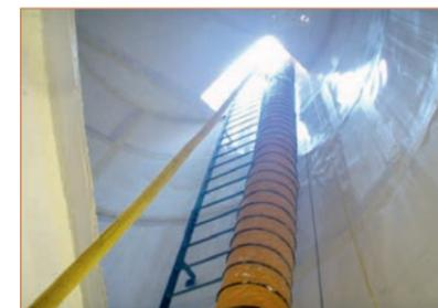
Photo 5 – View from the underside of a concrete platform within the drop structure after repair.
