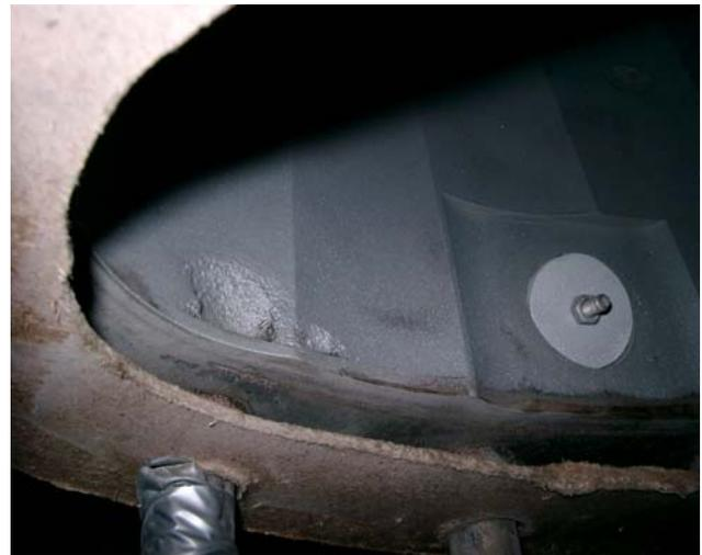
**Photo 6-SSE Forging-galvanic corrosion**
