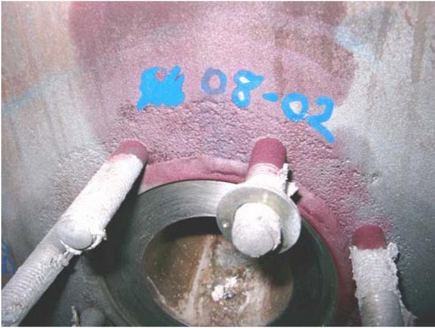
**Photo 3- Body End Valve- bolted joint**
