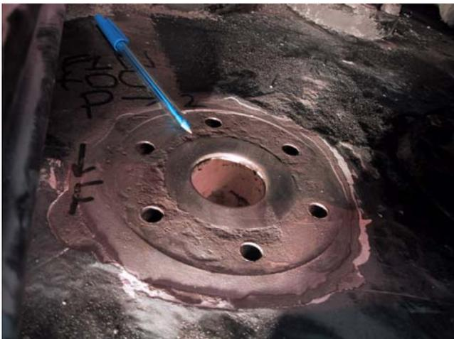
Photo1- Electrical Hull Penetration -bolted joint
