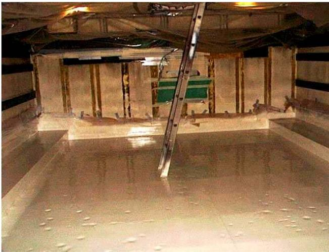
**Photo 5- Battery Compartment- pitting corrosion**
